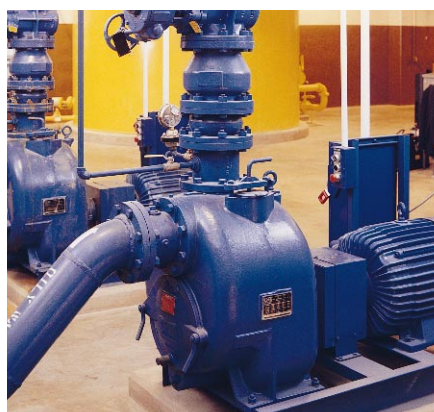
6" T Series™ pumps handling solids-laden wastewater at an automotive plant in Michigan, USA.
