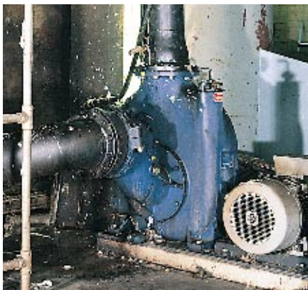
10" T Series™ pump handling abrasive run-off at an insulation factory in Norway.
