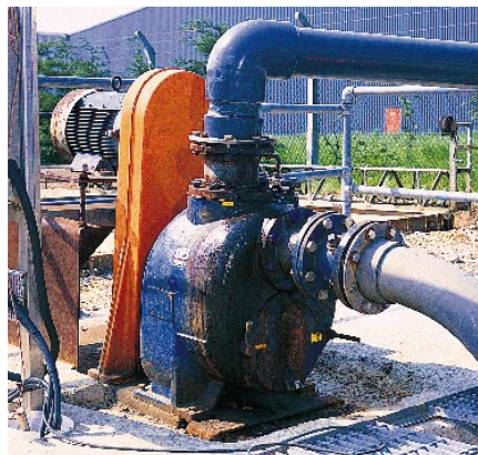
4" T Series™ pump handling corrosive wastewater at a pickling plant in England.
