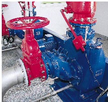
10" T Series™ pumps handling sewage at a treatment plant in Denmark.
