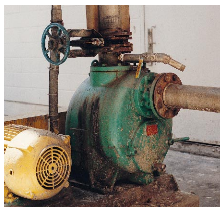
6" T Series™ pumping corrosive petroleum wastes at a waste recovery plant in the Netherlands.
