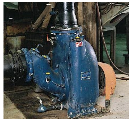
10" T Series™ pump handling abrasive, solids-laden run-off at a steel mill in Pennsylvania, USA.
