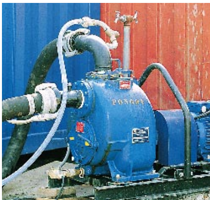
3" T Series™ pump handling wastewater at an automotive plant in Ohio, USA.
