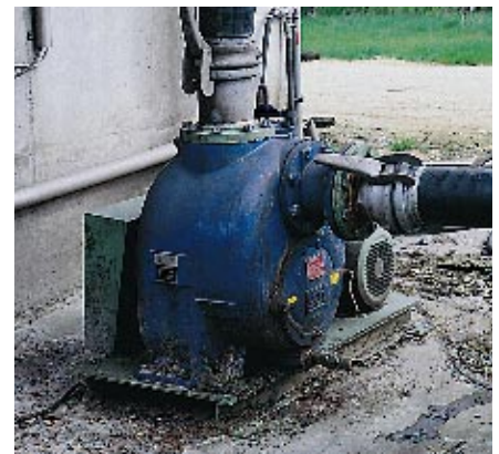
4" T Series™ pump transferring wastewater to a holding tank at a starch plant in Denmark.
